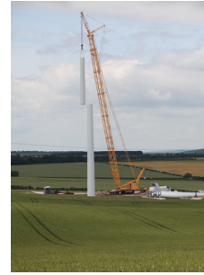
1. The lower sections are connected together
