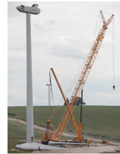
2. The hub and nacelle are put in place.
